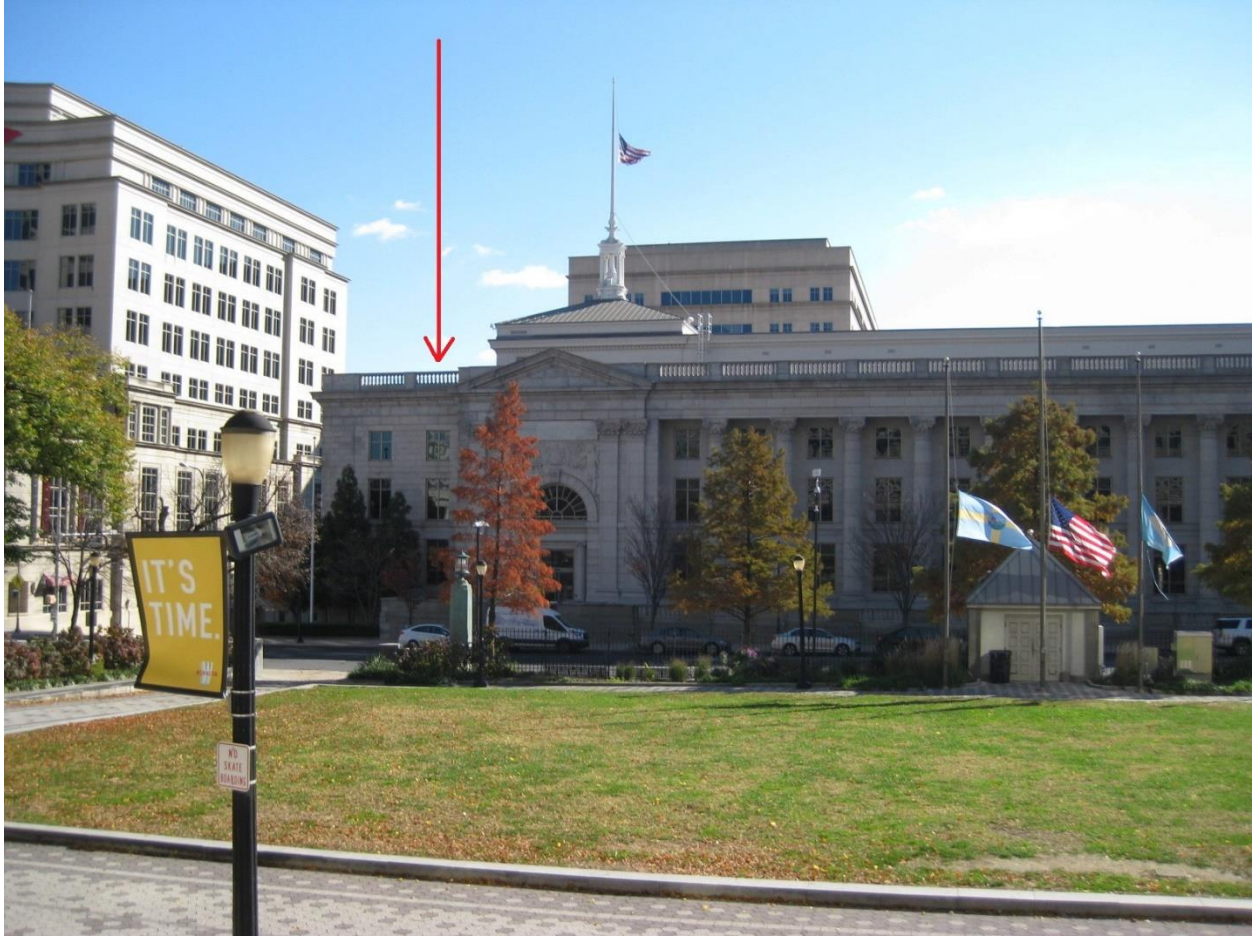
November 2018 view of the 1916 Public Building from the west in Rodney Square. The red arrow marks the approximate location of the old Strangers Burial Ground, which was removed to Wilmington and Brandywine Cemetery in the early 1850s.
